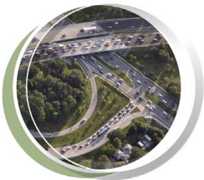
Congestion at the SR 13 / I-295 Interchange
