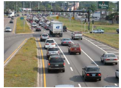
Congestion at US 17 / I-295 interchange
