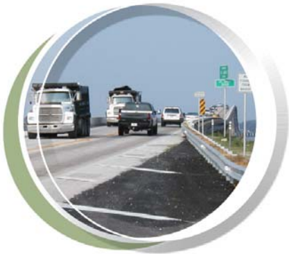
Traffic on the existing Shands Bridge
